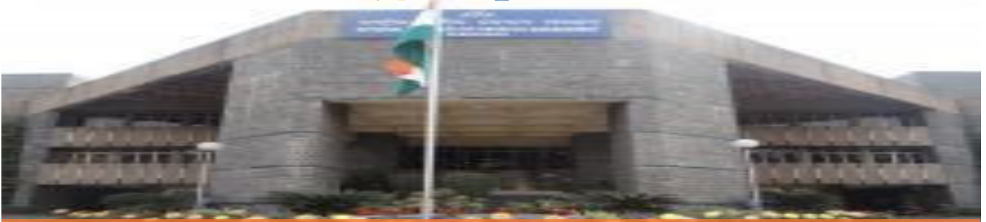
Main Building of AJNIFM
